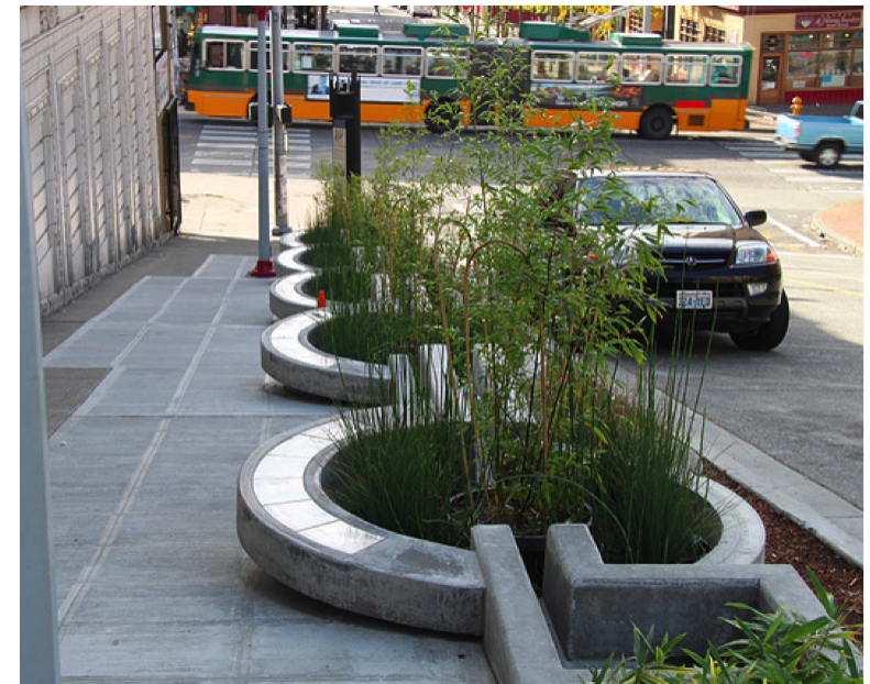
Figure 49: Stormwater Planter Source: http://www.southsidegreen.com/green-infrastructure-primer/
