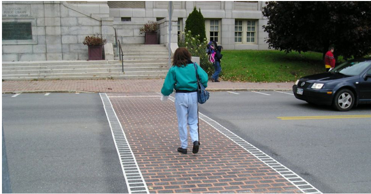
Figure 70: Crosswalks with alternate paving materials (Institute of Transportation Engineers, 2010)
