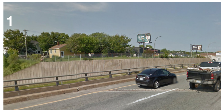
Figure 99: Existing Retaining Wall Highway 111 Exit Source: Google Maps Street View, 2015.
