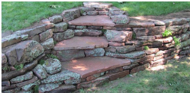
Figure 57: Stone steps and stone retaining wall built into hillside Image Source: http://stoneandturf.com/build-a-bench-or-stairs-out-of-stones-and-rocks/
