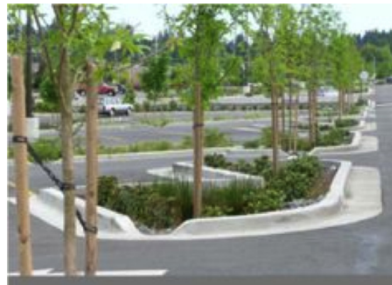
Figure 51: Curb Elimination in Parking Lot Source: https://www.pinterest.com/pin/510454938987467328/
