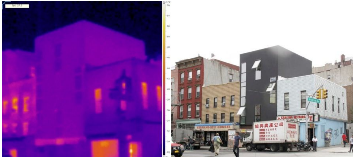
Williamsburg, New York, mixed-use Passivhaus apartment has superior heat retention compared to neighbours. 18
